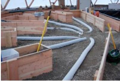
The rock/clay soil does not provide good drainage, so a drainage system is provided in all growing beds, consisting of 4" flexible corrugated pipe with holes, then covered with a sock to keep the holes from clogging. These pipes converge in the center, then go outside to drip into the future orchard area.
